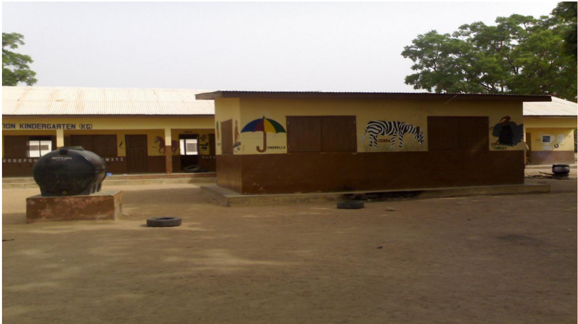
Figure 5.3: A school Building Constructed by Plan Ghana
