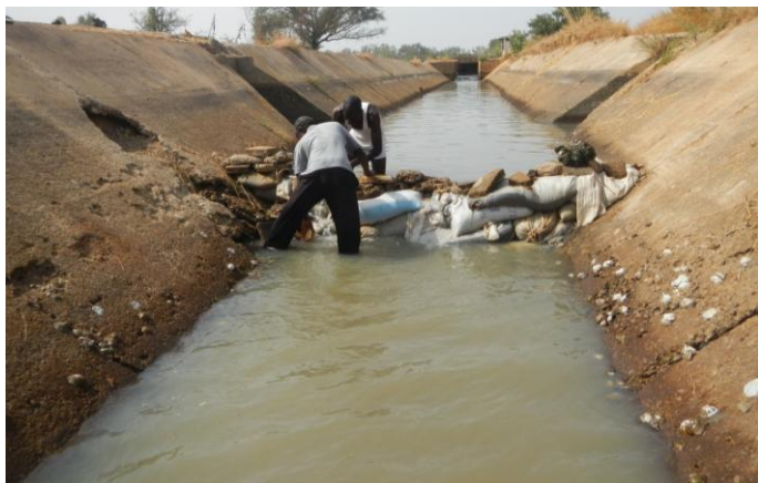
Plate 9: Farmers Improvising Check Structure on a Canal Using Sandbags and Stones in Tono Irrigation
