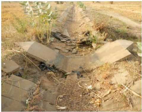
Plate 1: Conditions of Laterals in Tono Irrigation Scheme
