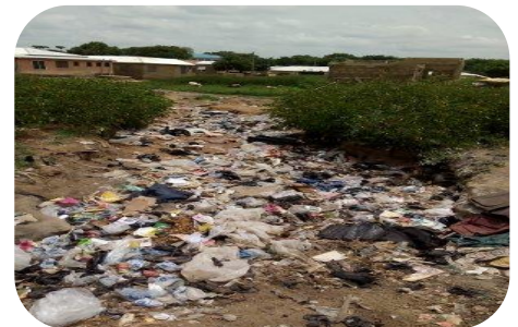
Plate 4.10: choked gully
