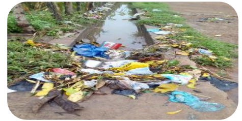
Plate 4.8: choked gutter
