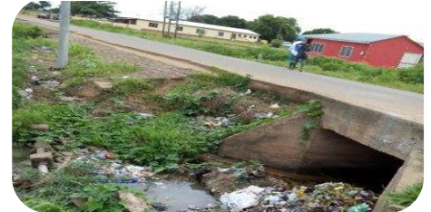
Plate 4.9: choked culvert
