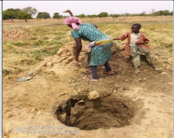
B -Manually refilling hand-dug well
