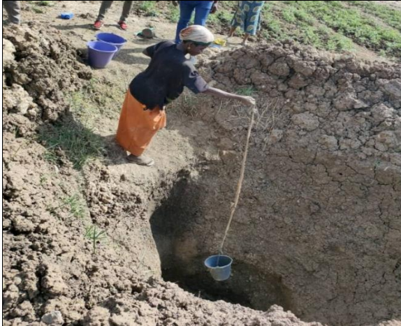
A- Manually abstracting water from hand-dug well
