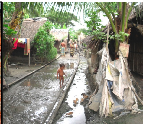
Fig. 4 – Poor conditions of access road; Location: Montu Colony, Khulna city
