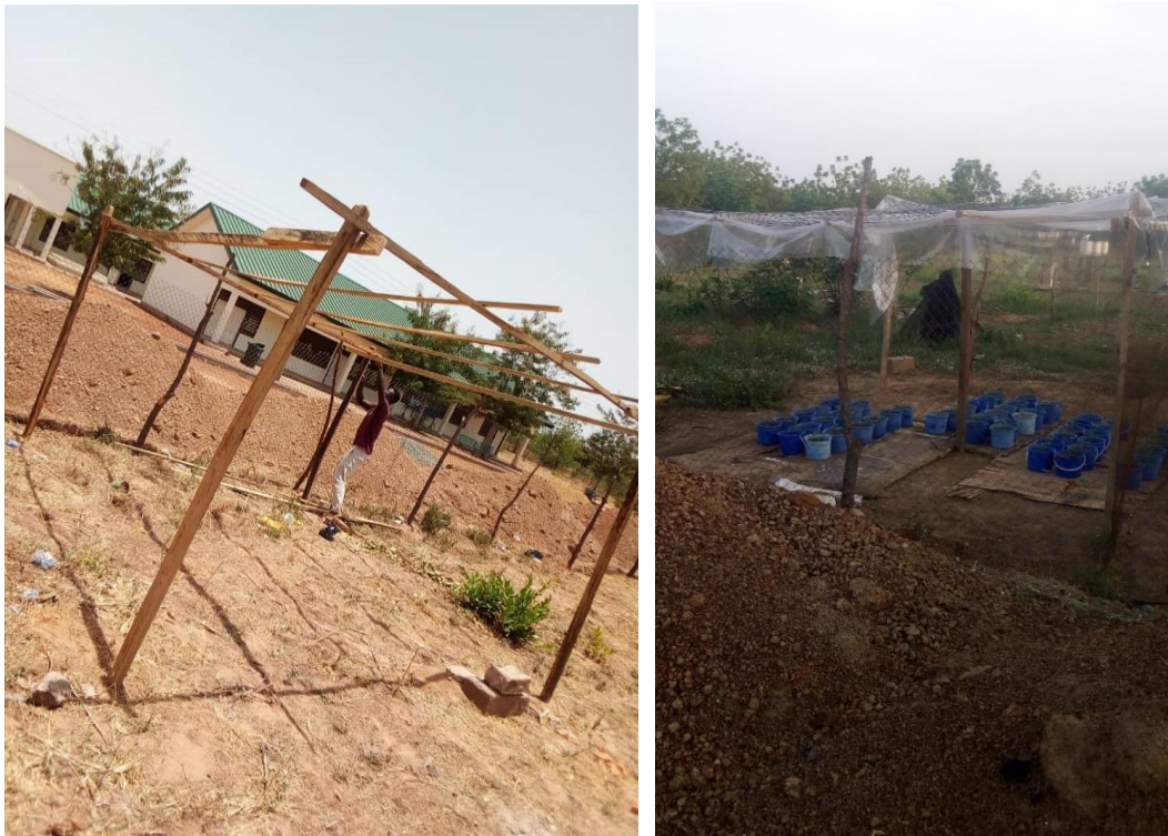
Plate 1: Construction of screen house
