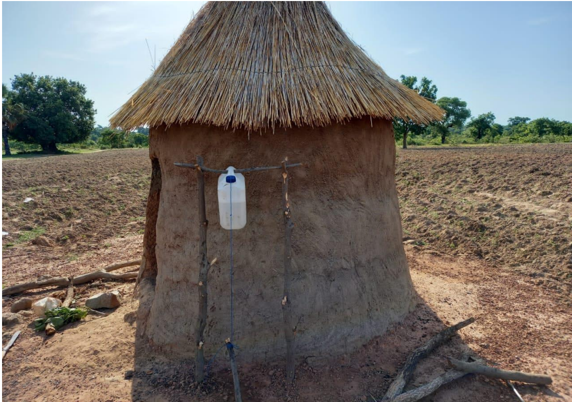
Plate 1: Local materials used to construct household latrine with tippy-tap for handwashing
