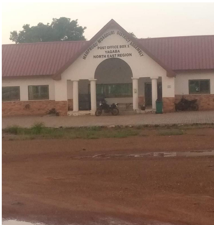
Photograph 1 Mamprugu Moagduri District Assembly Office
