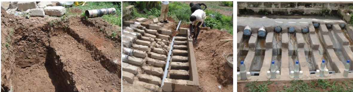
Plate 5.2: Constructional Process of Experimental Set-up in the Field
