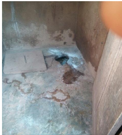
A KVIP household toilet facility in Worizehi
