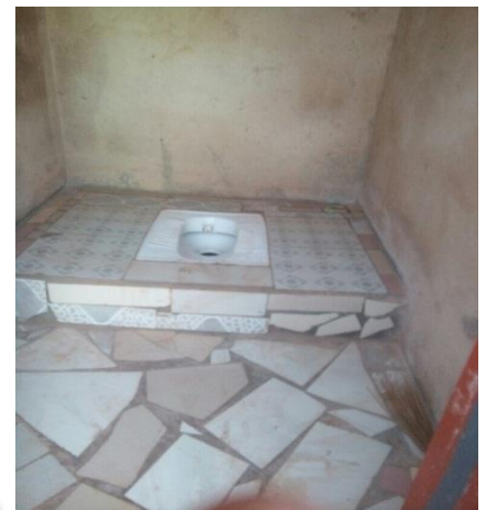
A Pour to flush household toilet facility in Gumbihini
