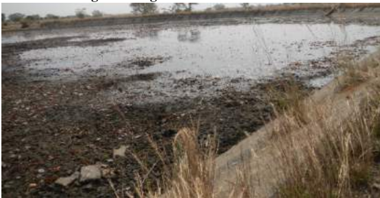
Plate 5: Silted Night Storage Reservoir 5 in Tono
