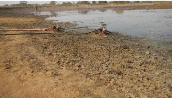
Plate 3: Silted Night Storage Reservoir 3 in Tono
