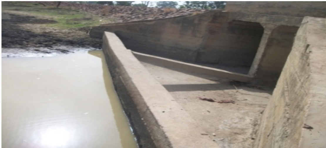
Plate 4.10 A typical Culvert Diversion in Kunyukuo
