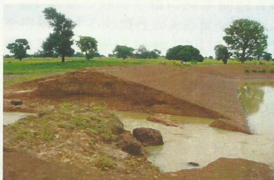
Photo 4. Break of Dam 4 wall
