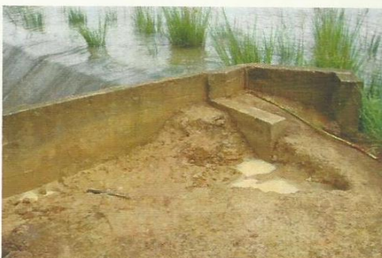
Photo 3. Eroded side of Dam 3 spillway
