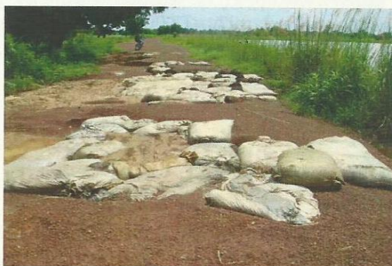
Photo 2. Protection of overtopped Dam 1 wall
