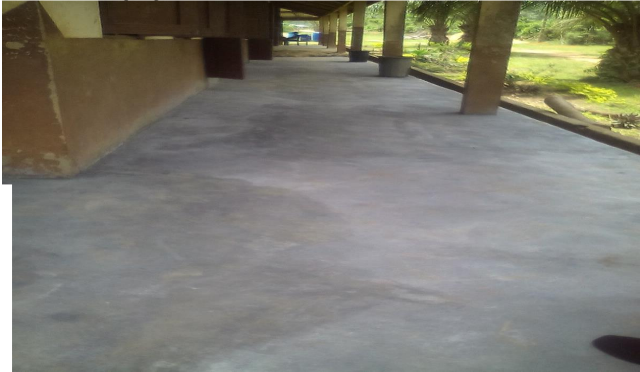
Plate 4. 5: An Ongoing Classroom Block Renovation at Asikam
