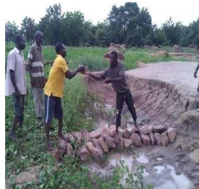
Plate 6.3a stone bond with grass re-enforcement, plate 6.3b gully erosion control
