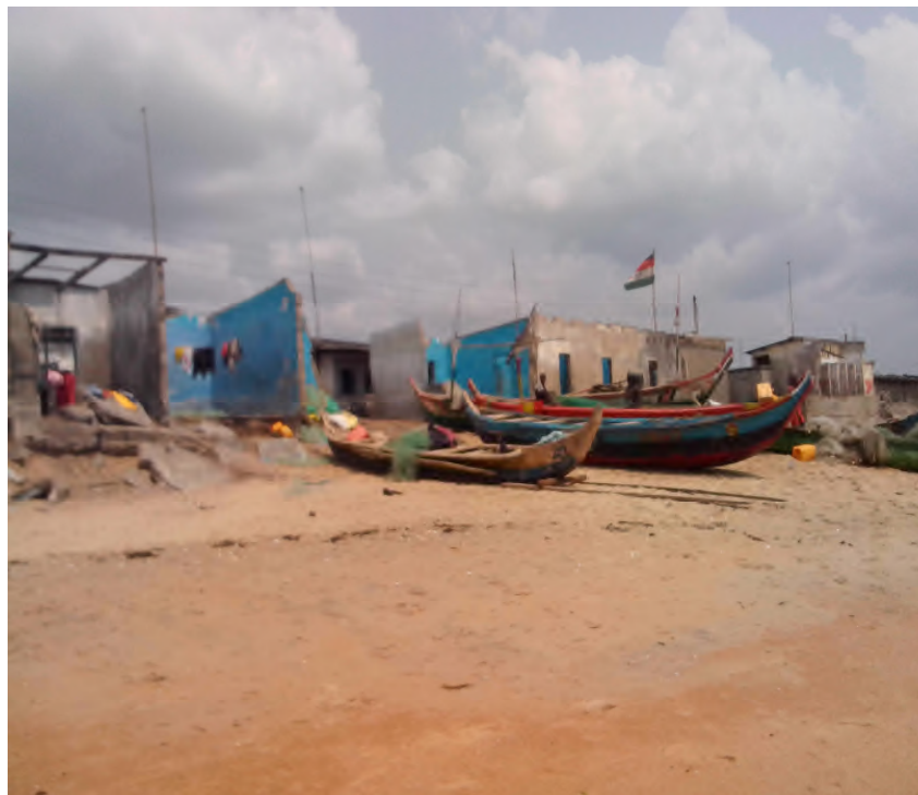
Figure 4.10a: Buildings affected by sea inundation at (Dutch) Komenda
