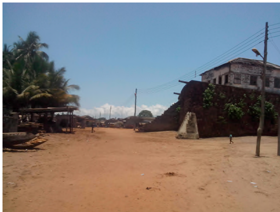
Figure 4.13: Defunct Fort (with plants on the wall) and other local structures at (British) Komenda
