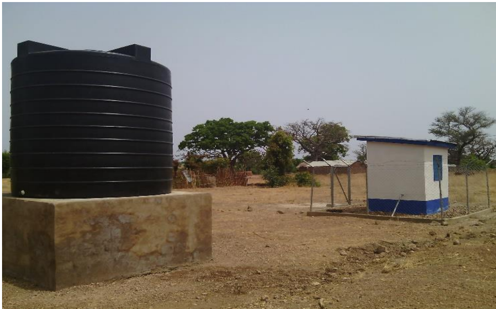
Plate 2 Overtank that supplies water to MUS points
