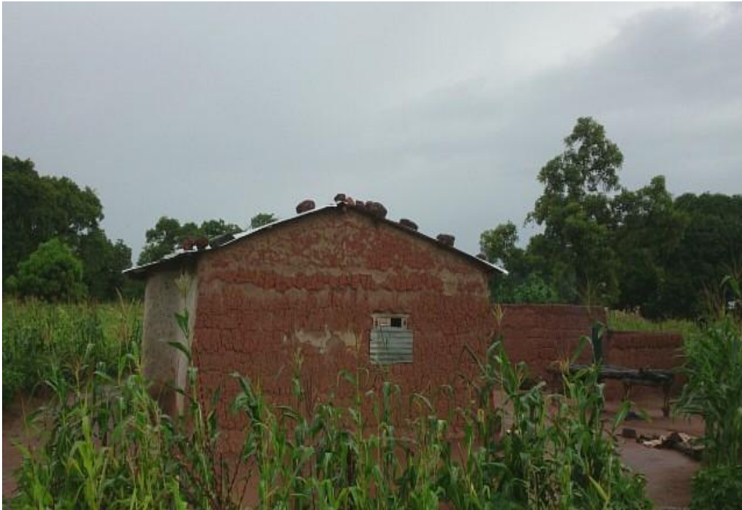
Figure 5. Picture depicting stone bonding to prevent destruction by rainstorm (Source: Fieldwork, 2014)
