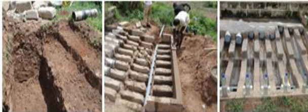
Plate 2: Construction Process of Experimental Set-up in the Field
