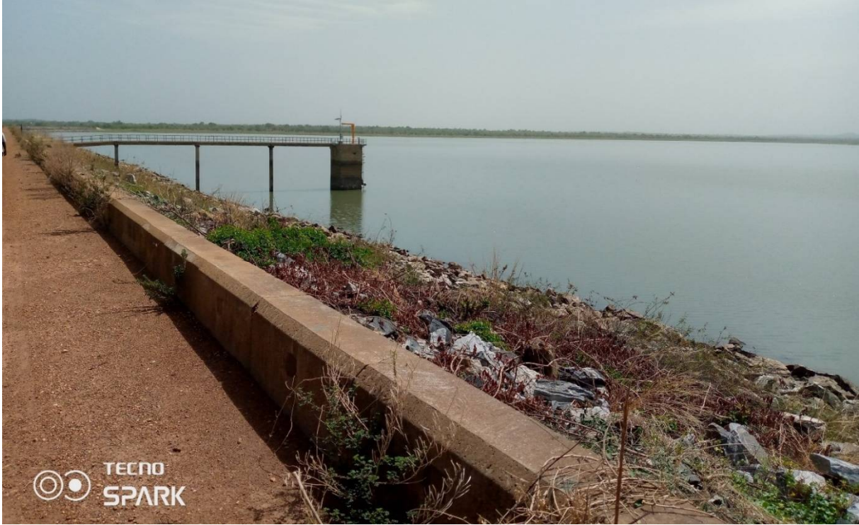
Figure 1: Tono Irrigation Dam
