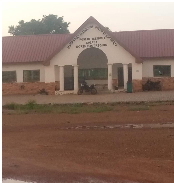
Photograph 1 Mamprugu Moagduri District Assembly Office
