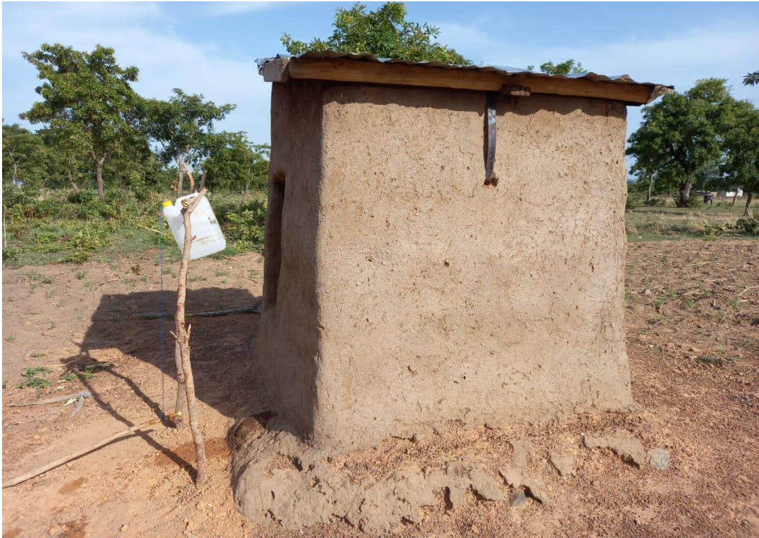
Plate 2: The use of local and some improved materials for household latrine construction with tippy-tap for handwashing.
