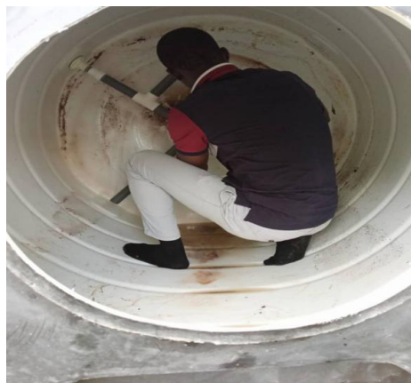
Fixing of PVC pipe distribution network system in filtration tank
