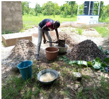
Washing of filter material
