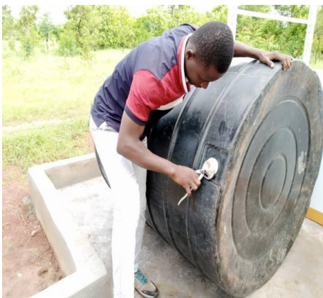
Tighten of poly tank connectors
