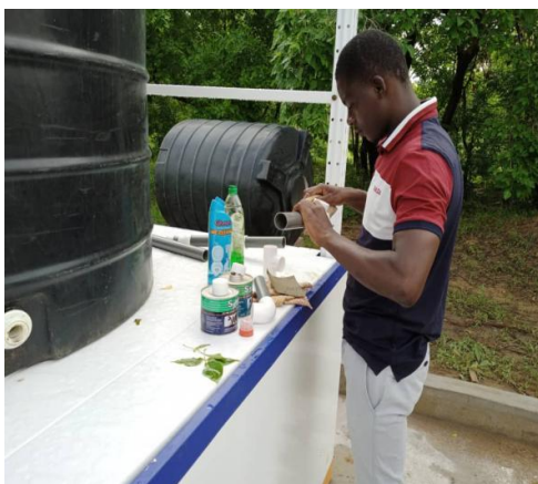
Fixing of PVC elbow
