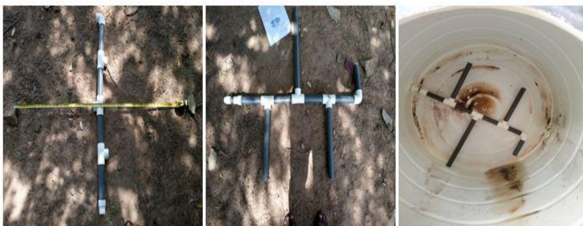
Figure 3.3: Inner View of the Inlet Pipe (Left) and Inlet Pipe Network (right)
