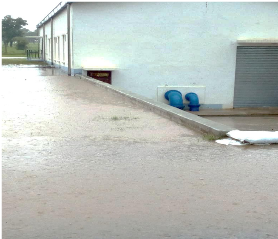
Plate 4.3: Water on some parts of the facility
