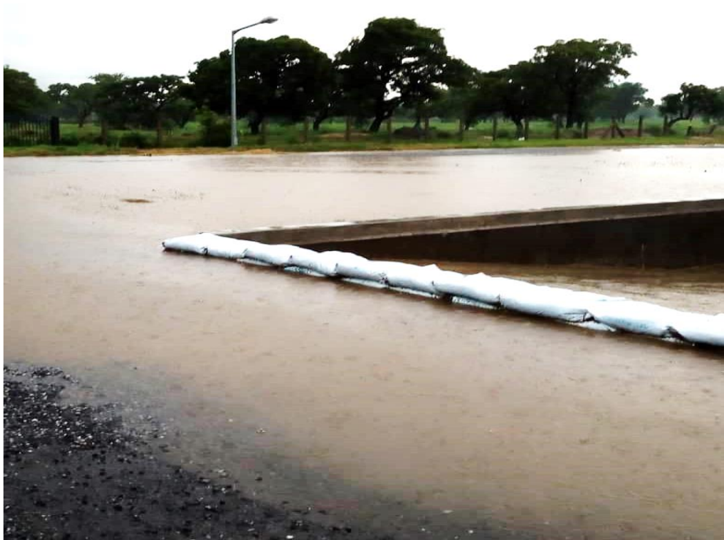
Plate 4.2: Rainwater just at the verge of the facility
