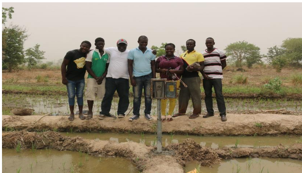
Figure 3.6: Installing time lapse camera in zone H of the Tono Irrigation Scheme
