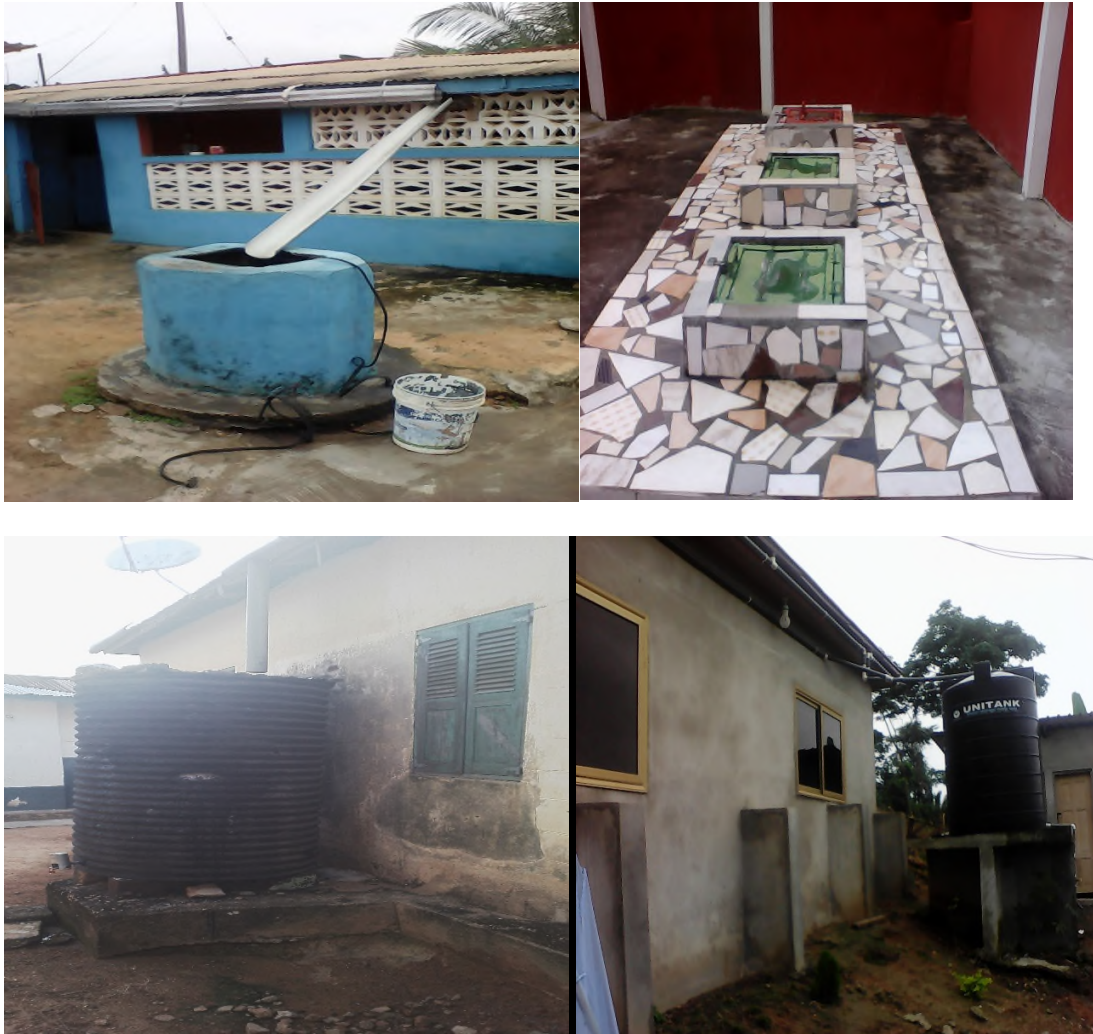
Figure 4.3 Storage Devices for Harvested Rainwater in the Assin South District.
