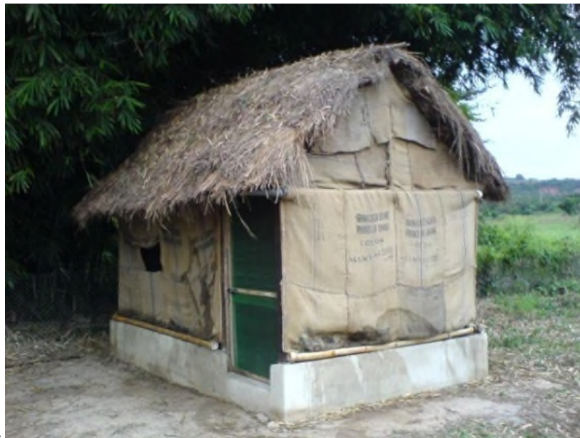
Plate 1: Evaporative cooling barn (Source: Teye et al. , 2011a)
