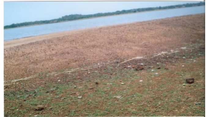
Plate 2: Pile of sediments in the Vea reservoir 33 years after construction
