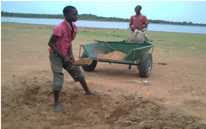
Plate 4: Sand winning in the Vea reservoir for the purposes of construction
