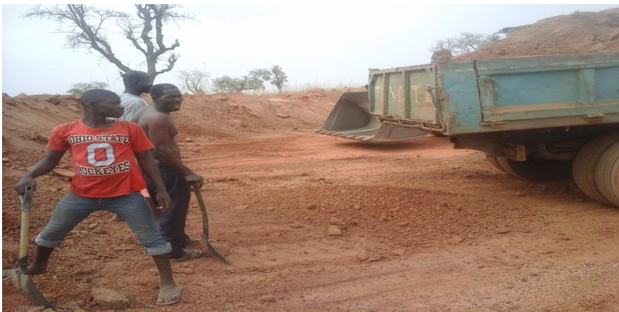
Image 4.4 Shows some gravel loaders with shovels at work.
